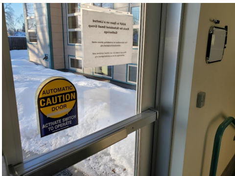
Automatic door openers installed on both south doors.
