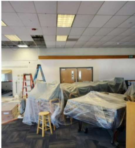
During Construction: Removed wall was on the left by the ladders.
