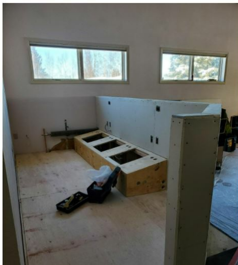
A/V Control Booth partly built.
