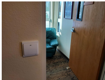
New light switch
