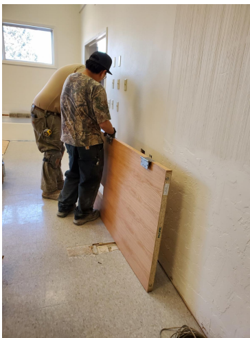
Preparing to install new doors.
