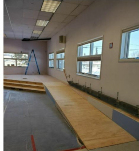
Ramp and stairs are built. Ready for carpet and railing.
