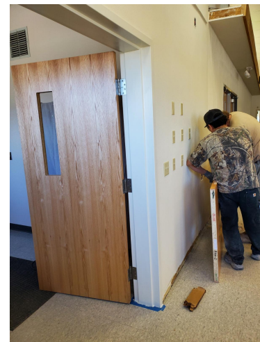
New doors installed.
